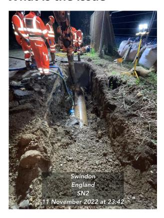
The pipe is a 500mm diameter GRP (Glass Reinforced Polymer) pipe.
